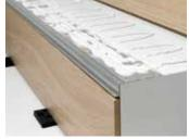
Apply glue to the sub-profile and the step. Spread the glue out across the sub-profile.
