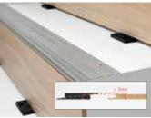
Glue the plank to the riser with Quick-Step One4All glue. The spacers ensure that sufficient space is left underneath to fit in the next step.
