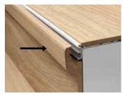
Press the Incizo® profile onto its sub-profile and position it nicely for a level transition with the rest of the tread. Repeat the installation for the rest of the stairs.
