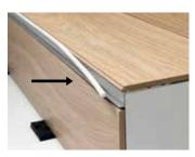
Place a plank on the step against the rising edge of the sub-profile. Push the plastic strip\* on the tongue of the plank.
